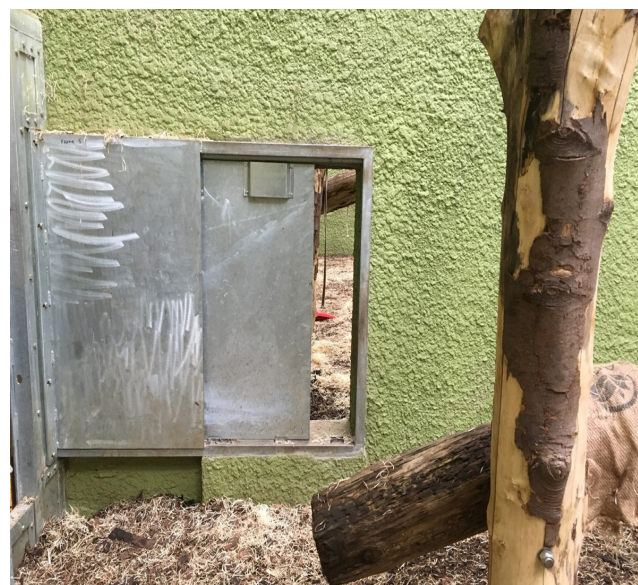
Figure 1. Shows the 'creep' as a narrow gap that enables female individuals to pass through into the other half of the enclosure, but not a large male. The sliding door used was always locked securely into place on its runner.
